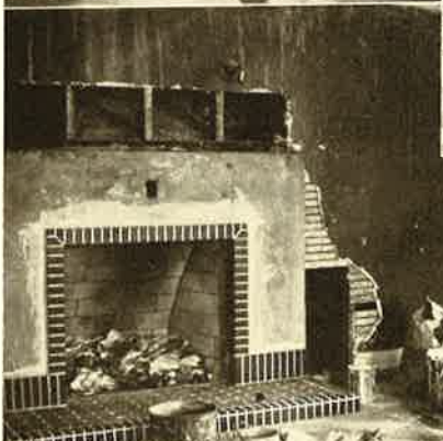
SENIOR ROOM FIRE-PLACE IN THE MAKING
